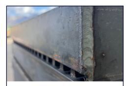
Trench Banding elevates the banding bar for efficient drainage, keeping liquids from being trapped between the band bar and the embed angle.
