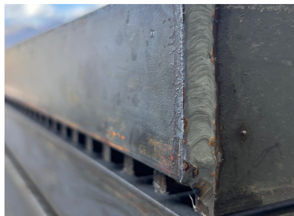
Trench Banding the grating by elevating the banding bar for efficient drainage that will not trap liquids between the band bar and the embed angle.
