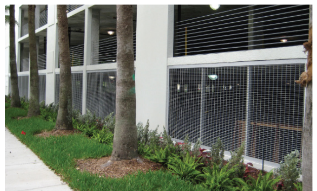
Ground floor security/ventilation screen
