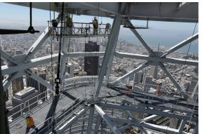
The tallest building in California at the time of construction, Interstate Gratings built each piece of grating for the Transbay Sales Force Tower in San Francisco. The streets had to be shut down for each delivery so the material could be lifted via crane to the top of the building. The complicated details, such as layout challenges and multi-angled sections, were fabricated with accuracy which allowed the grating platform to be utilized during construction.
